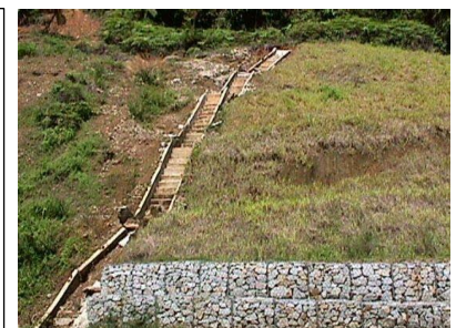
Figure 4: Cascade drains
