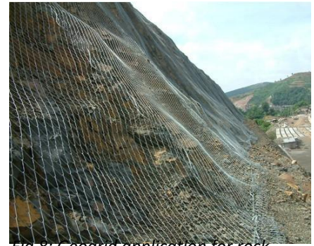
Fig 8: Geogrid application for rock fall protection: http://rockfallmesh.sell.everchina.com/p-
