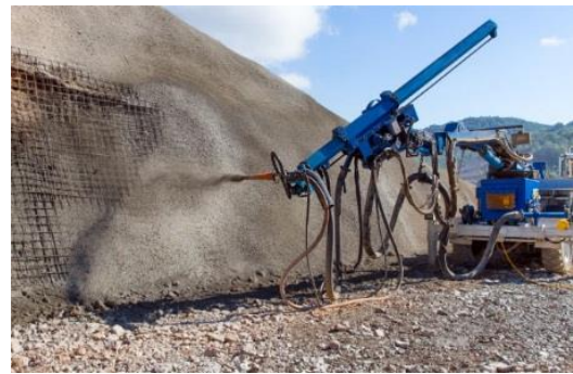
Figure 11: Shotcreting of slopes
