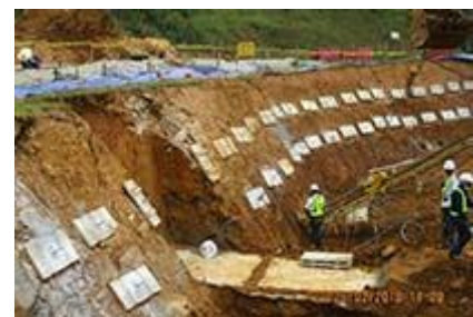
Figure 7: Rock bolting: RDA SL
