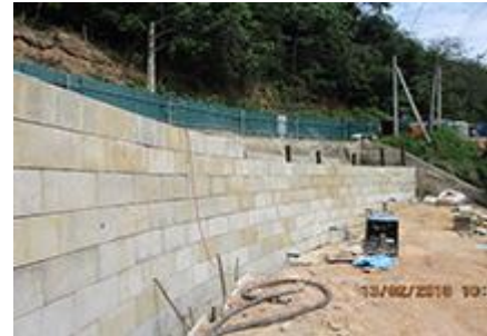
Figure 8 : Retaining wall: RDA SL
