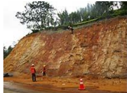
Figure 3: Modification of slope geometry: RDA SL
