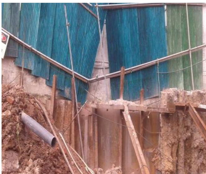
Figure 01: Effect of inadequate support system to neighboring structure.
