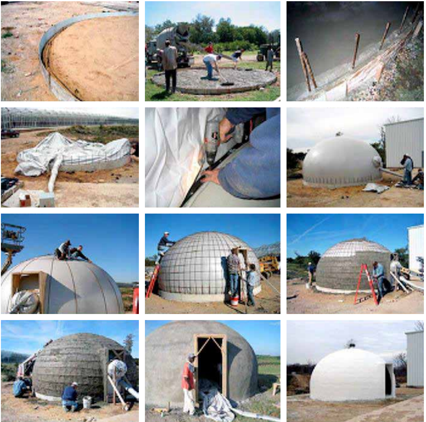
Figure 01: Dome house construction process (Source – Hammer, C. (2006). Optimization of Dome Housing in Sri Lanka)
