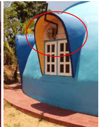
Figure 05: Covered the area allocated for permanent ventilation by using temporary materials.
