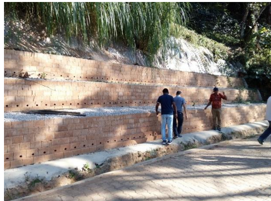
Participants inspecting the mitigation completed by “TOR” blocks
