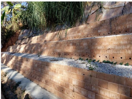
Participants inspecting the mitigation completed by “TOR” blocks
