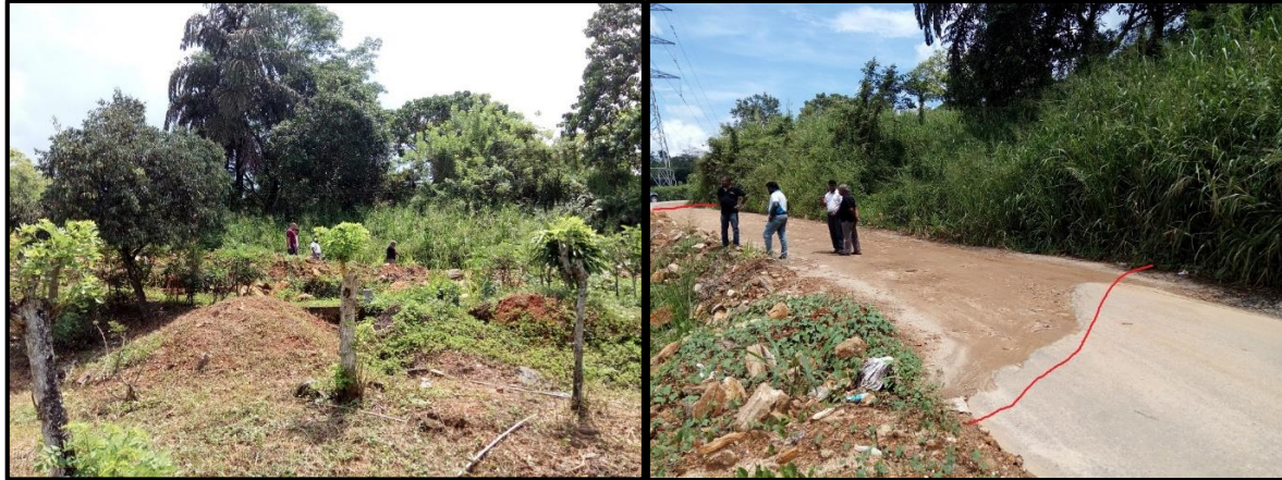
Few photos of Project team carrying out field investigations at site
