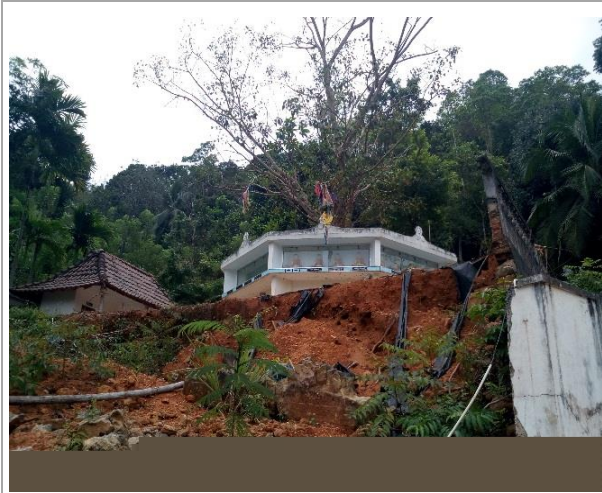
Fig 2a: Cutting failure near the Bhoodhiya
