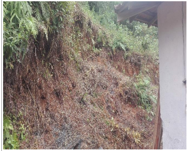
Fig 2b: Area of cut slope behind the hermitage.
