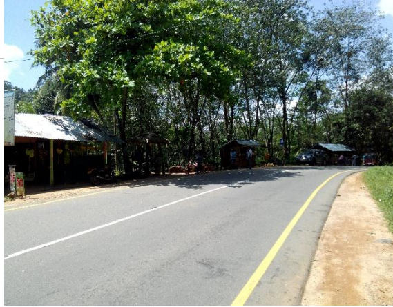
Fig a: Current appearance of the road bend in landslide area
