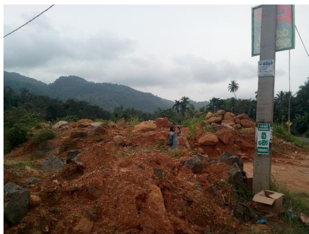
Fig e: Rock boulders and mud deposited on down slope area.
