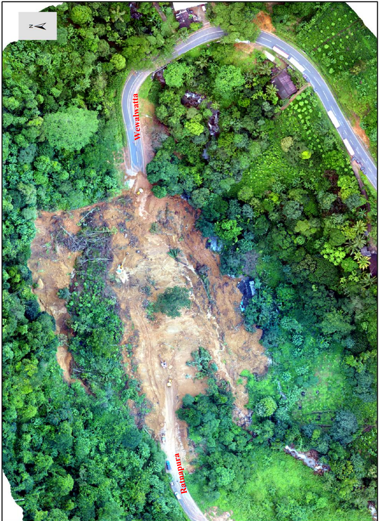
Annexure I: Drone image of the project area (soon after the failure)
