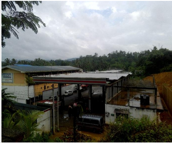
Fig 2a: Filling station in front of the landslide
