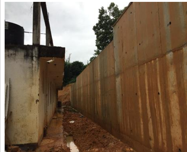
Fig 2c: Retaining wall built by the land owner as a temporary measure
