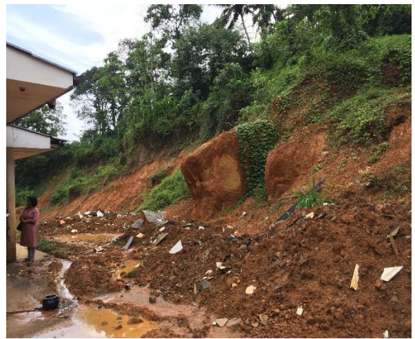
Fig 2d: Deposition of the mud and rock behind the damaged house.
