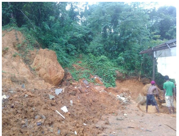
Fig f: Damaged up slope area
