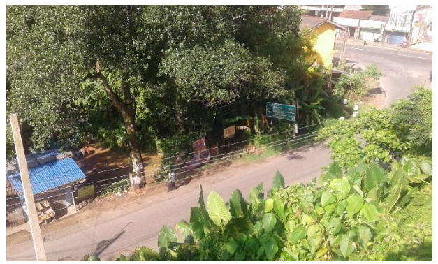
Fig 2b: Downslope view of the slope failure from the school side
