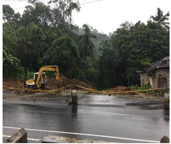
Fig 2b: RDA remediation works on the already moved downslope (09-08-02018)
