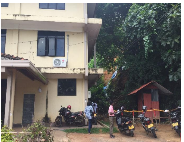
Fig 2f: District Labor Office building at risk (downslope)
