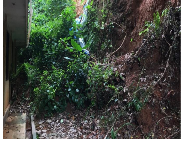
Fig 2b: The passage between the failed slope section and the Labour Department building where debris had deposited due to the incident
