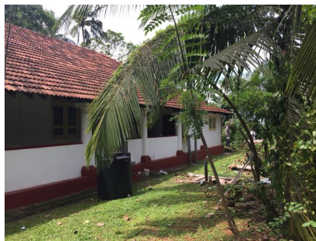
Fig 2e: Hermitage of the Sudharshanaramaya at risk (upslope)
