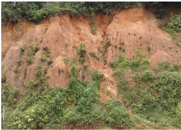
Fig 2c: Upslope of the road. Section between 4/4 & 4/5
