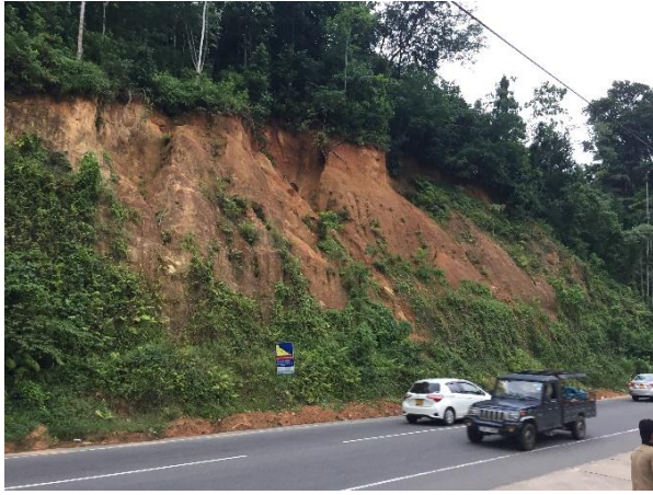
Fig 2a: Upslope of the road. Section between 4/1 & 4/2
