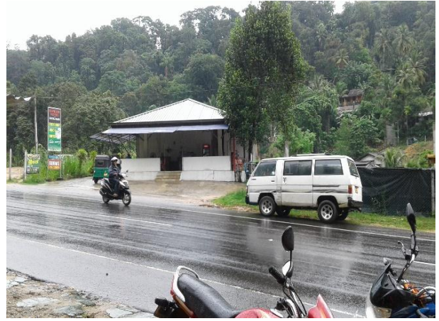
Fig 2b: Downslope of the road, section between 4/1 & 4/2
