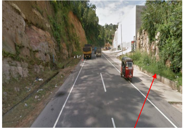
Fig 2d: Downslope of the road, section between 4/4 & 4/5
