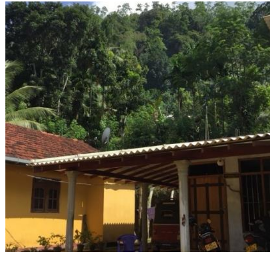
Figure 4: House in potential slope failure area
