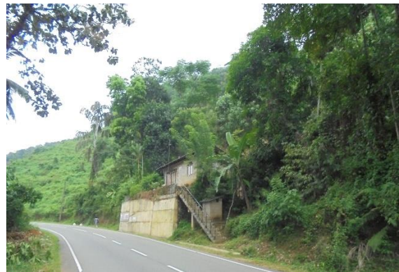
Fig d: The medium risk home located upslope
