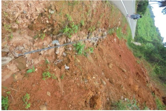
Fig 2c: Water line runs at the toe area
