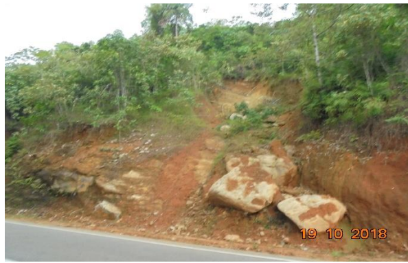
Fig c: Stones felt down with the slope failure
