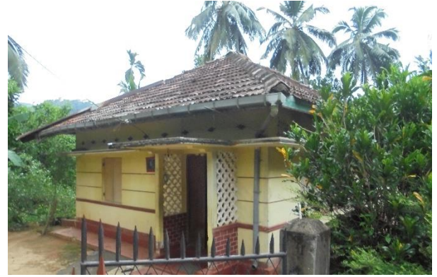
Fig 2d: Risk houses at the toe area
