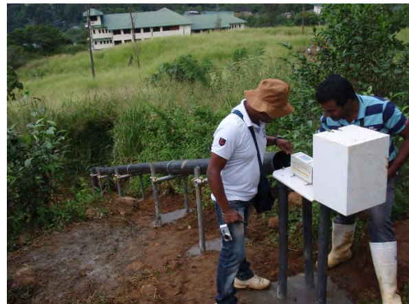
Installation of an Extensometer
