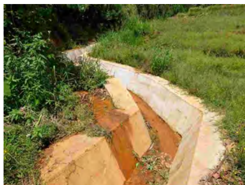
Smoothly modified ditch line
