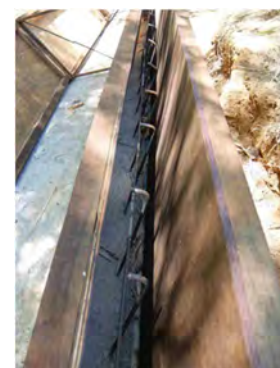
After restoration work
