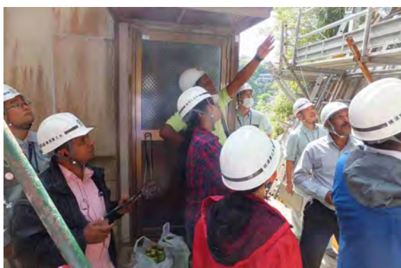
Countermeasure Work in Kanagawa Prefecture
