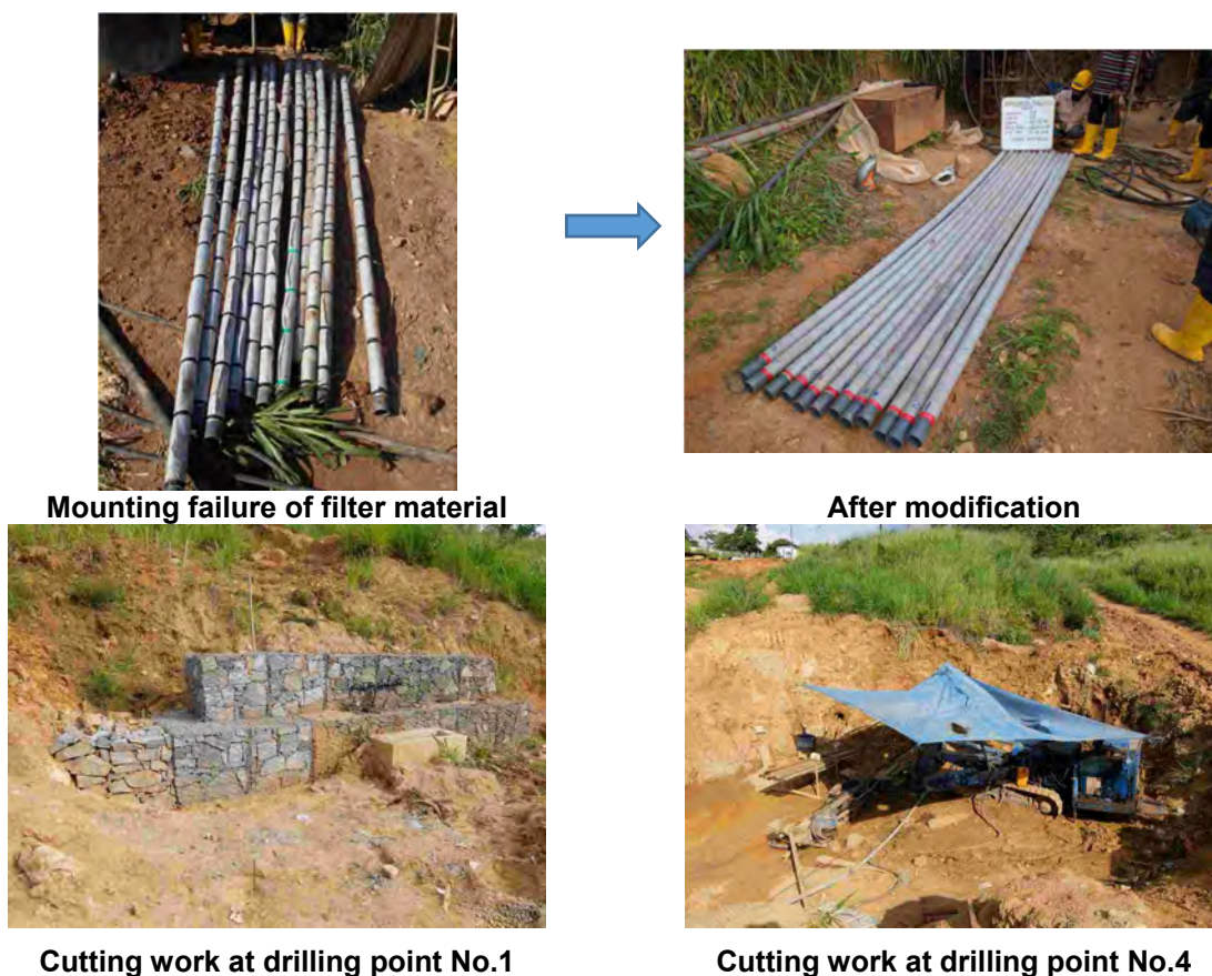
Photo 5.8 The Situation of Horizontal Drilling
