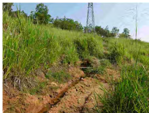
Springwater of drilling point at upper part of No.1
