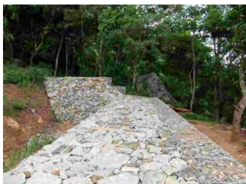
Surface of the embankment
