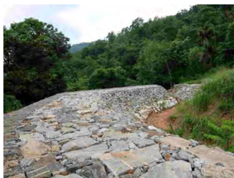
Surface of the embankment
