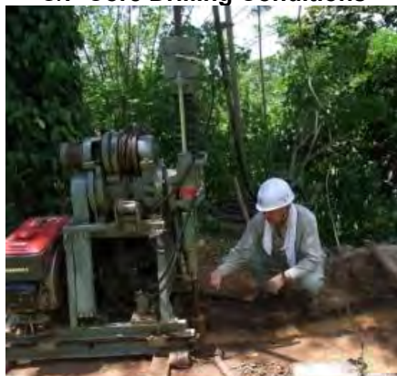
Core Drilling with a New Drilling Machine
