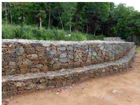
Front view of the embankment
