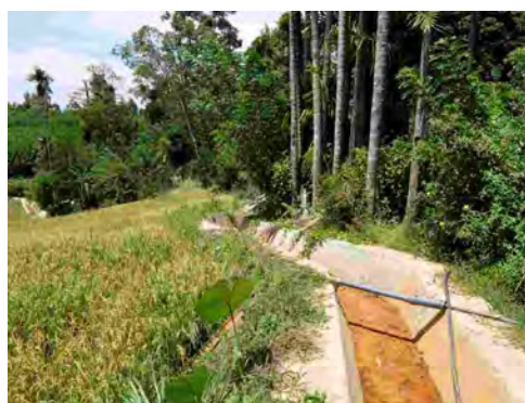
Smoothly modified ditch line
