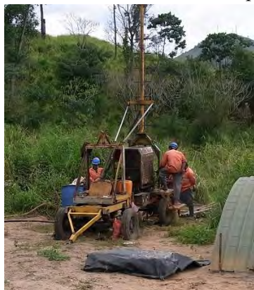
C/P Core Drilling Conditions
