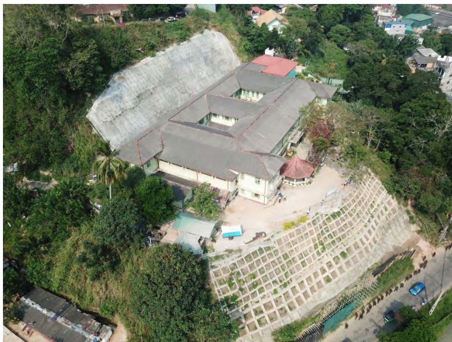
Photo 6.1 Drone view after construction (23th Mar 2018)
