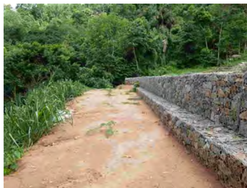
Front view of the embankment
