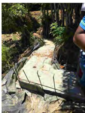
Ditch line turns almost at right angle
