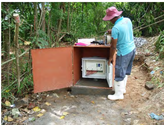
Installation of a Pipe Strain Gauge
