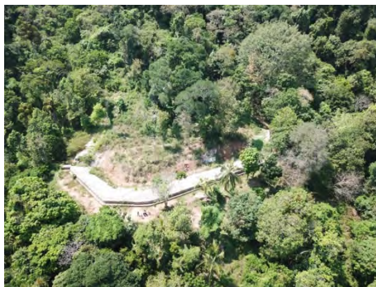
Photo 7.1 Drone view after construction (22th Mar 2018)
