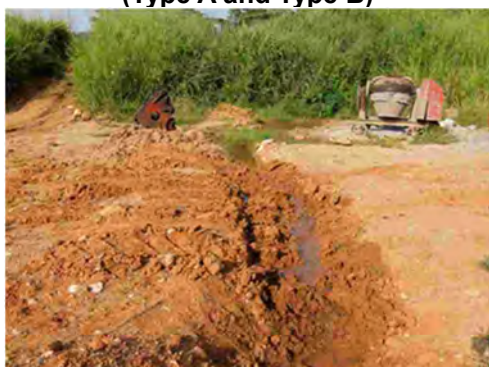
Springwater of drilling point at upper part of No.4
