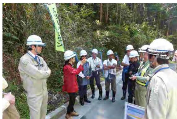
Countermeasure Work at Yui Landslide
