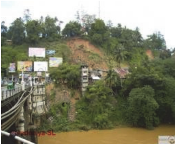
Figure 2-3: Slope failure occurred in Peradeniya
