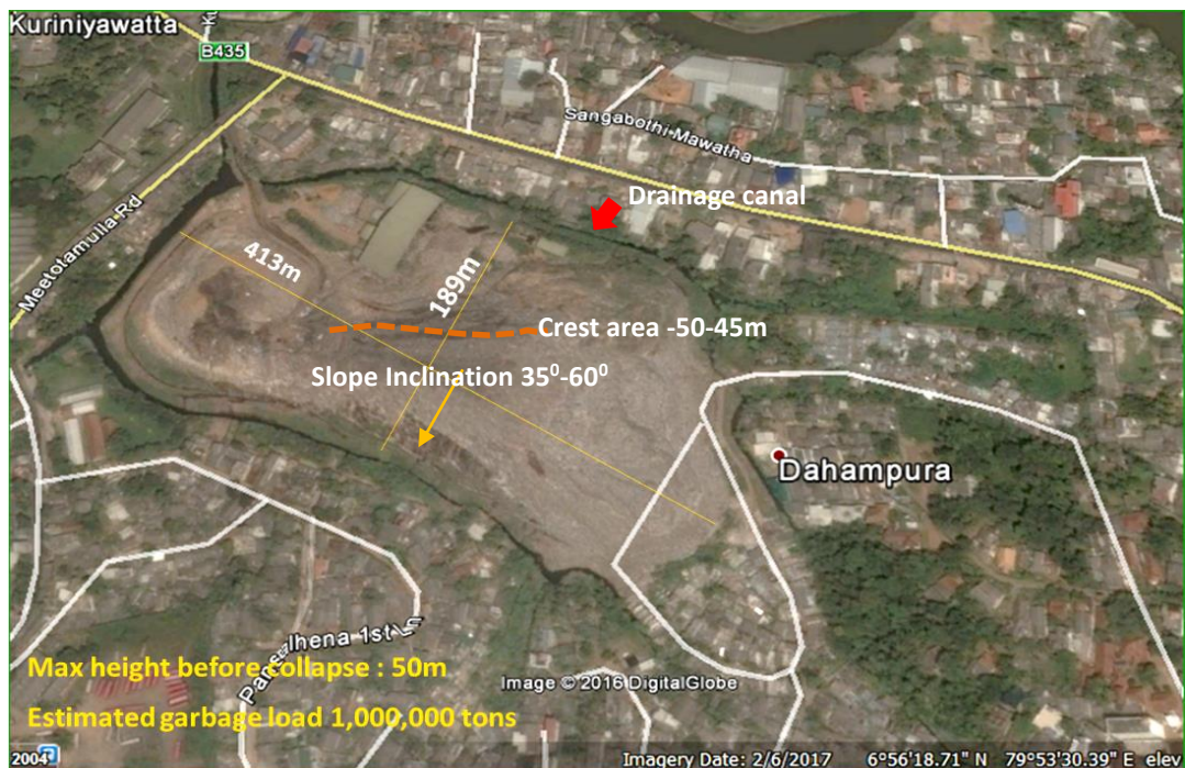
Figure 4: Spatial details of the Municipal solid waste dump in February 2017 before the collapse: Source: Google earth
